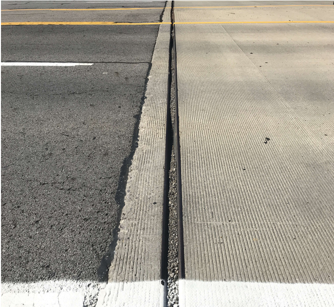
PHOTO 3 Description East abutment expansion joint assembly-Gravel accumulation.
