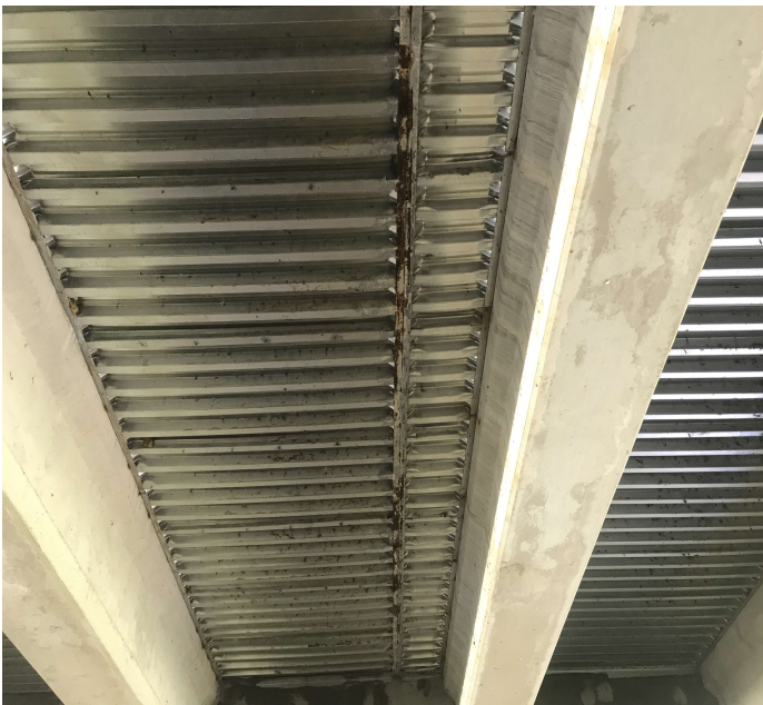
PHOTO 1 Description Corrosion to SIP forms along construction joint.
