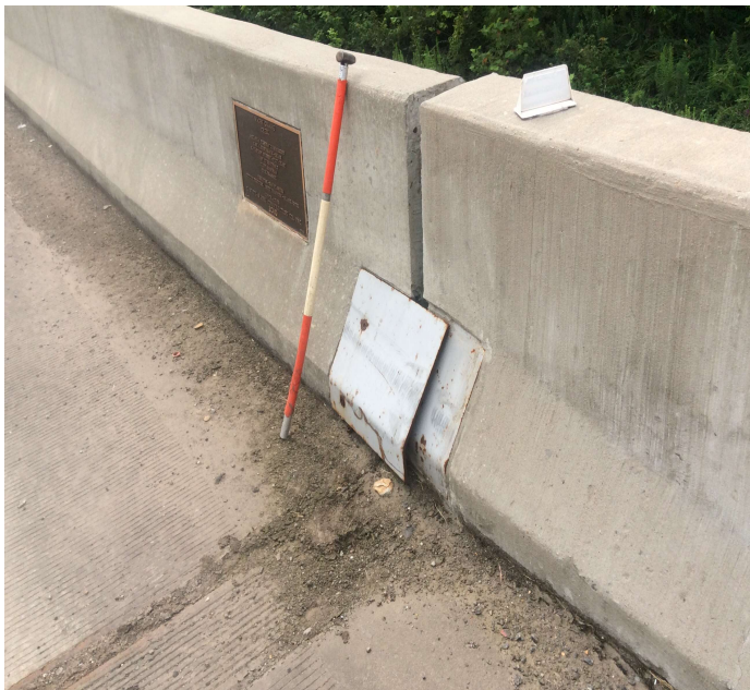
PHOTO 1 Description South sliding plate at Bent 1.
