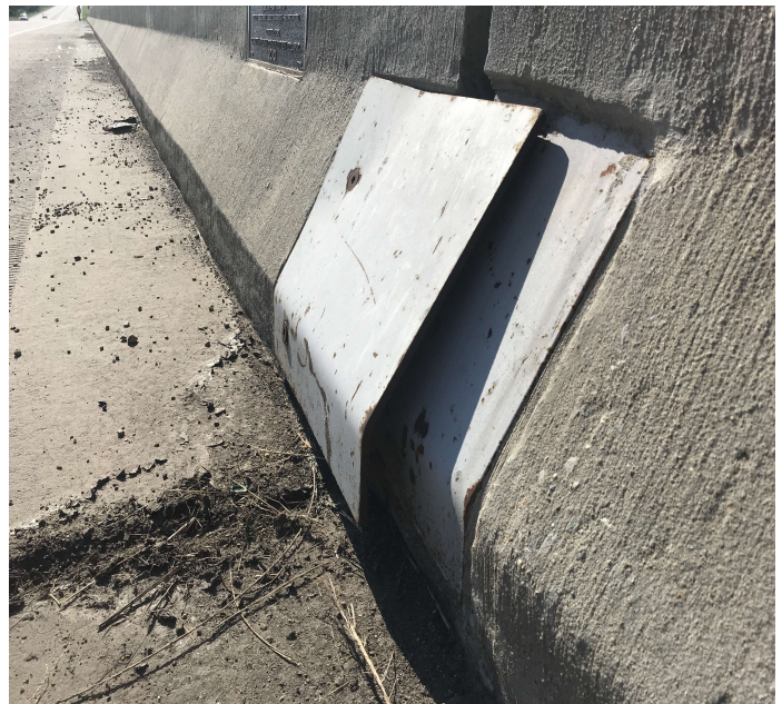
PHOTO 1 Description The steel cover plates attached to the right parapet wall have out of plane bending at Both abutment expansion joints.
