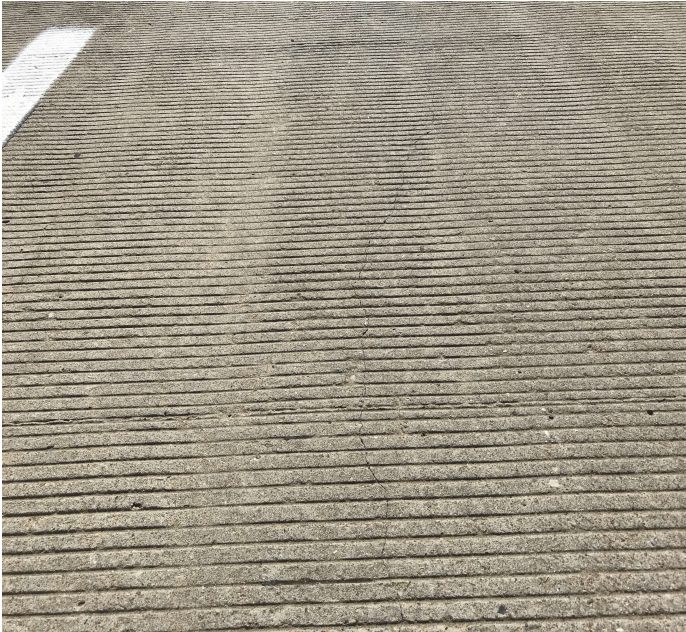
PHOTO 3 Description Longitudinal deck cracking.
