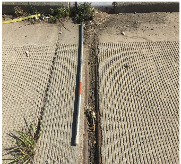
PHOTO 2 Description The expansion joints at both abutments have dirt, debris and gravel accumulation in the gutters and in portions of the driving lanes.
