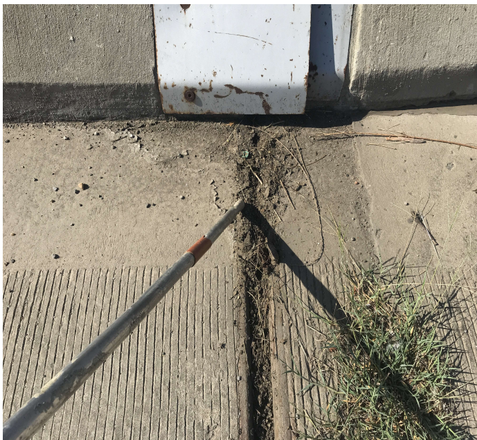
PHOTO 1 Description Dirt and debris expansion joint assembly.
