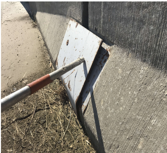
PHOTO 2 Description The steel cover plates attached to the right parapet wall have out of plane bending at Both abutment expansion joints.
