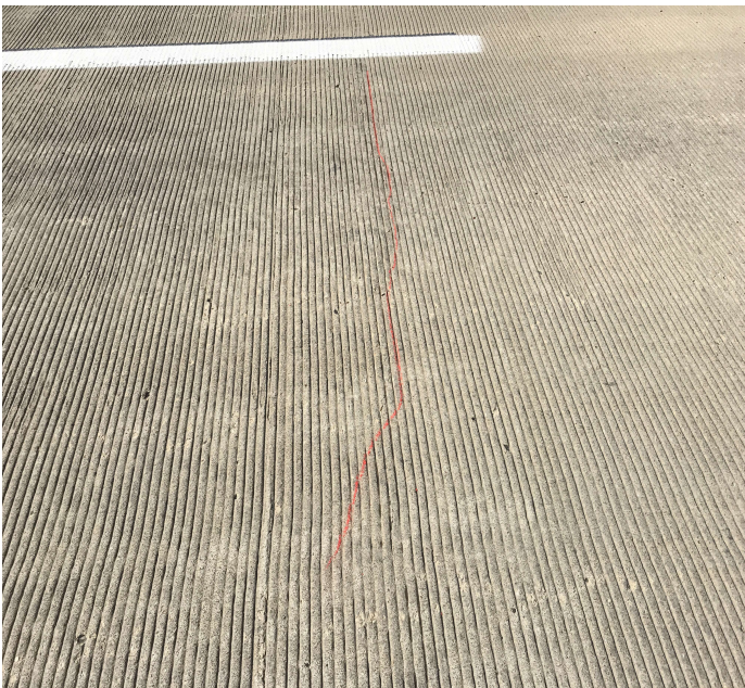
PHOTO 1 Description Transverse deck cracking.
