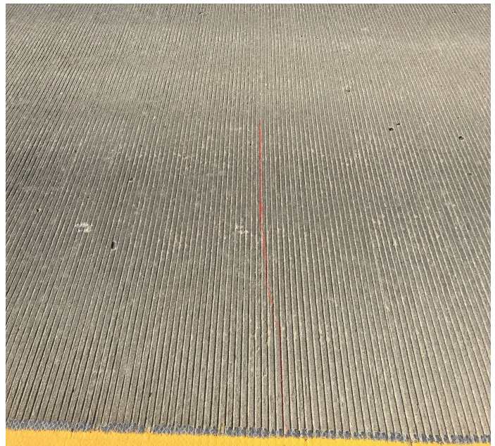
PHOTO 2 Description Transverse deck cracking.
